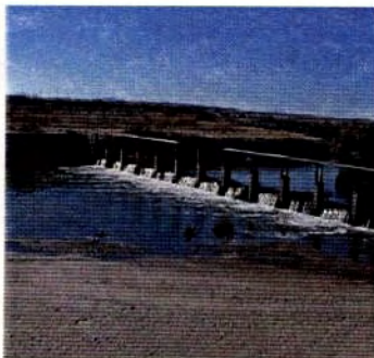
Station 15795 - Rio Grande at Alamo Grade control structure.
