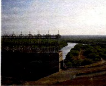
Power generating plants at International Falcon Reservoir
