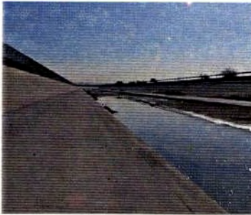
Channelized section of the Rio Grande (Segment 2308) in the El Paso area.
