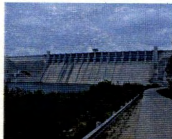
International Amistad Reservoir spillway
