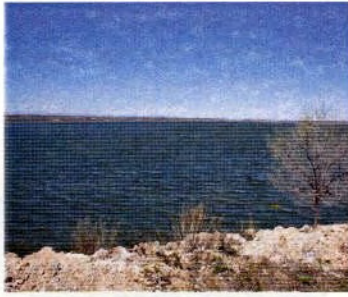
Red Bluff Reservoir from on top of the dam.
