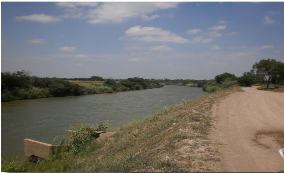
Pictured to the left is station 13177, Rio Grande at El Jardin Pump Station
