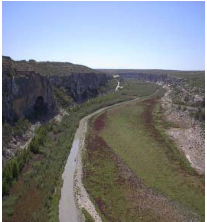
The Pecos River from the US90 bridge prior to the confluence with the Rio Grande.
