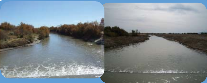
Station 15795 upstream of Fort Hancock, TX, before maintenance work (left) and after (right)
