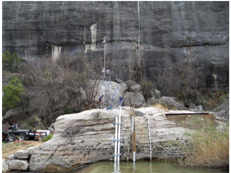
Installation of the CWQM station near Langtry TX
